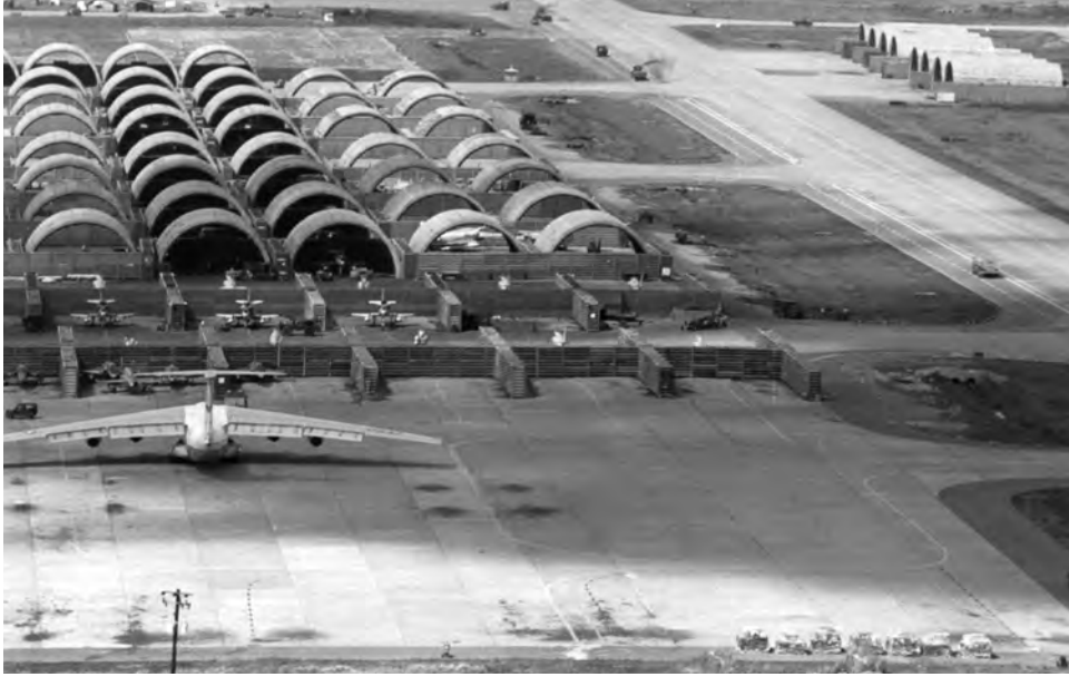
Wonder Arches like these at Bien Hoa Air Base could not be used for all types of aircraft, and the Army used less expensive revetments.
